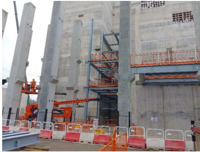
Figure 2: Billington, a subcontractor, continue IBA steelwork.
