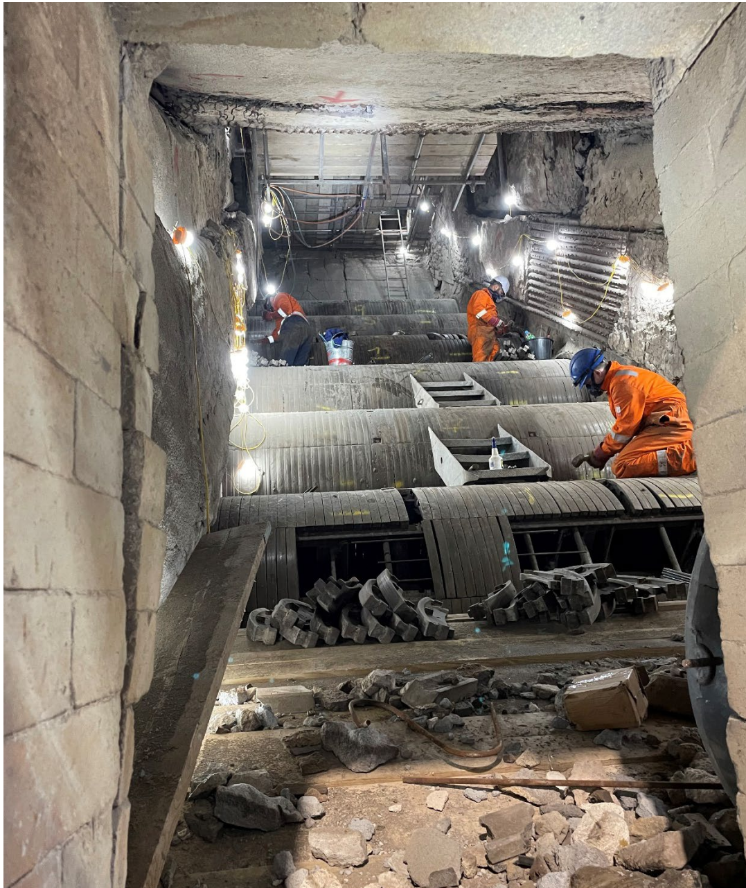
Figure 1: Planned outage works inside boiler 5, refurbishing of the roller gates
