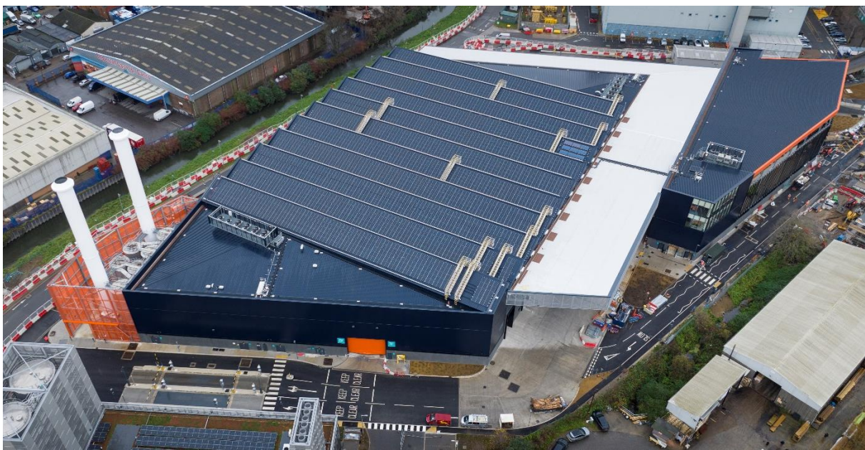
Figure 4: The Solar Array on the Roof on the RRF
