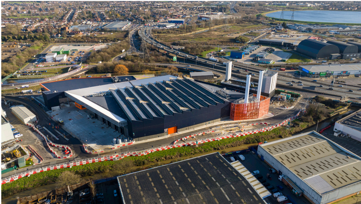
Aerial View of the completed Resource Recovery Facility ready for operation
