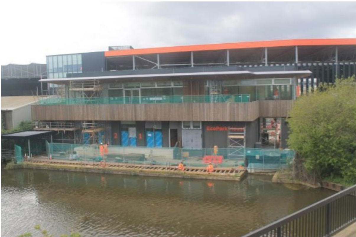
EcoPark House under construction
