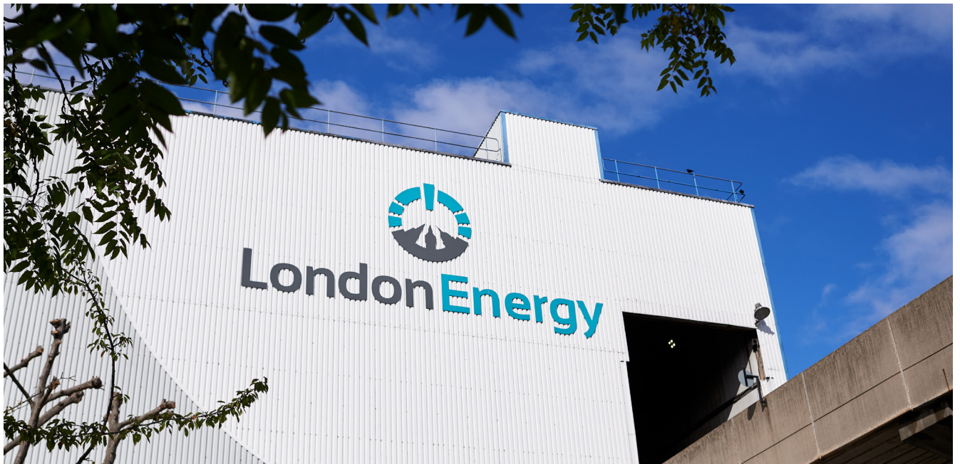
Energy from waste facility at Edmonton EcoPark
