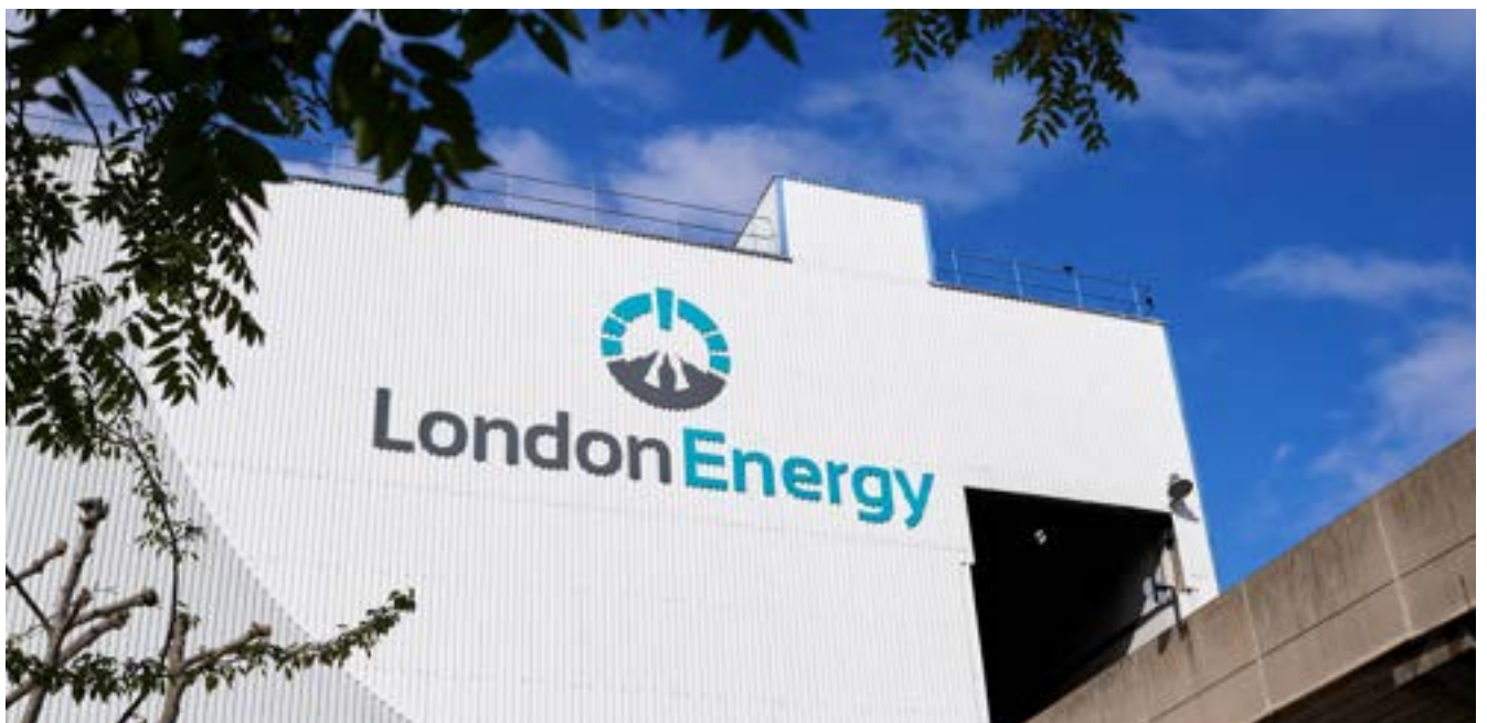
Energy from waste facility at Edmonton EcoPark
