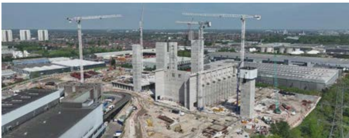
Aerial View of the ERF site under construction
