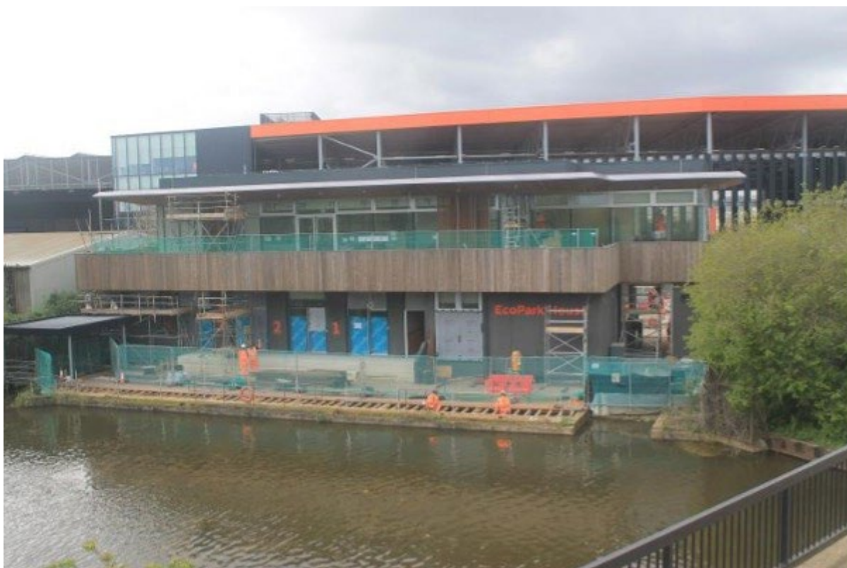
EcoPark House under construction
