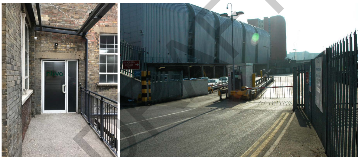
Berol House in Tottenham Hale and Hornsey Street Reuse and Recycling Centre in Islington
