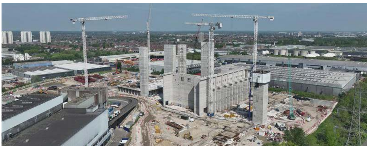
Aerial View of the ERF site under construction
