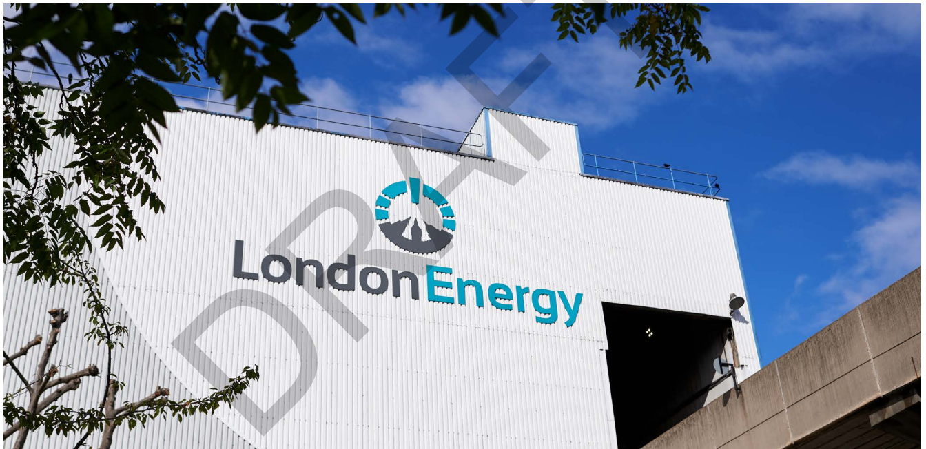
Energy from waste facility at Edmonton EcoPark
