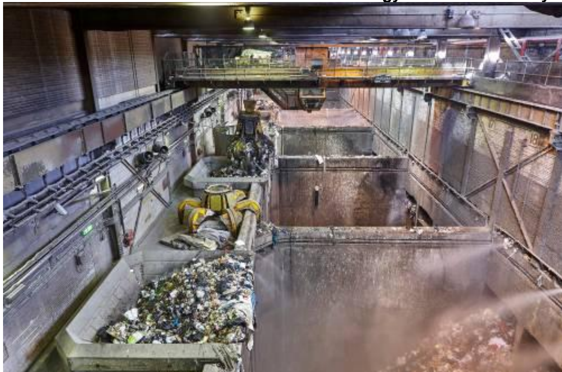
Photo 22.1: Waste bunkers at the Edmonton energy-from-waste facility
